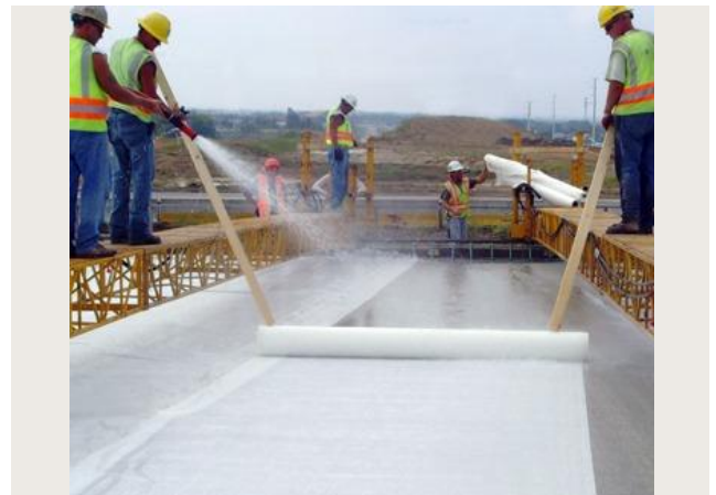
Figure 1-22: Proper curing is essential for concrete to reach its maximum potential for durability and strength.
