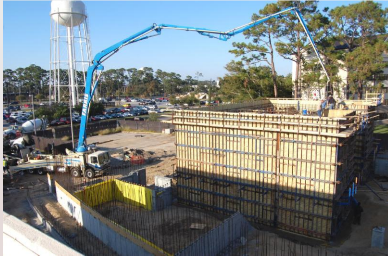
Figure 1-19: The mobile concrete pump is a very popular placement method
