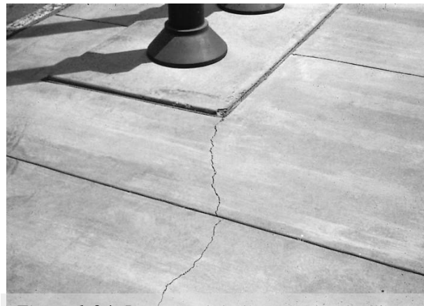
Figure 1-24: Improper jointing can cause unsightly cracking due to drying shrinkage. (Courtesy of Portland Cement Association)
