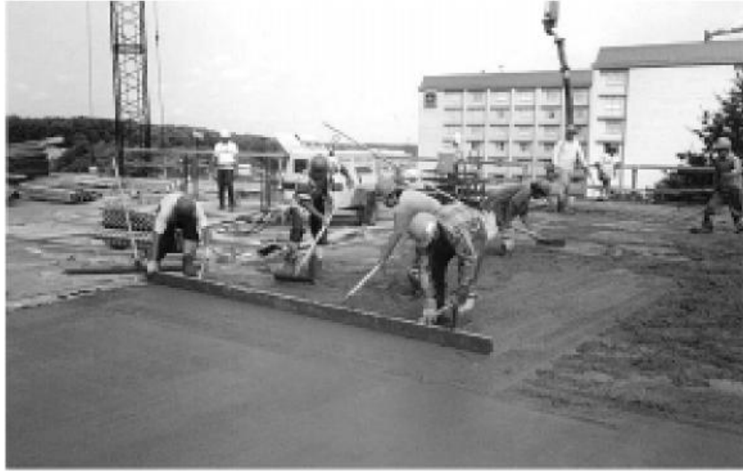
Figure 1-21: Proper timing and sequence of finishing operations is essential for quality flatwork.
