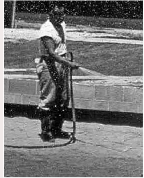
Figure 1-20: Subgrade should be slightly moistened in dry conditions. There should be no standing water on the subgrade before concrete placement. (Courtesy of Portland Cement Association).
