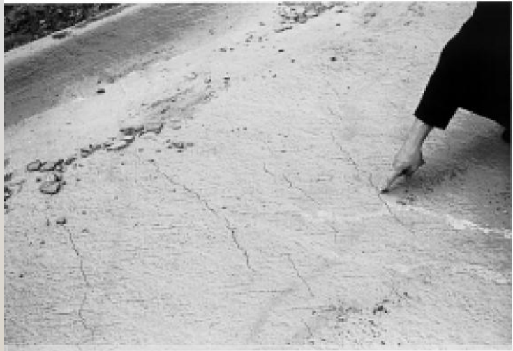
Figure 1-23: Plastic shrinkage cracking can occur if the surface of the concrete is allowed to dry out before the concrete sets. (Courtesy of Portland Cement Association).
