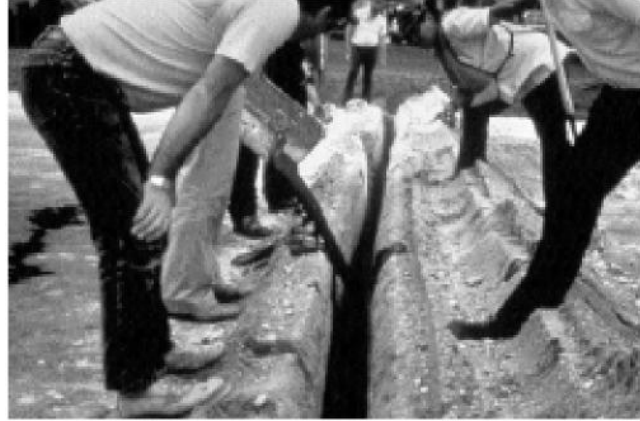
Figure 1-10: Flowable Fill (Controlled Low Strength Material) is an economic fill material
