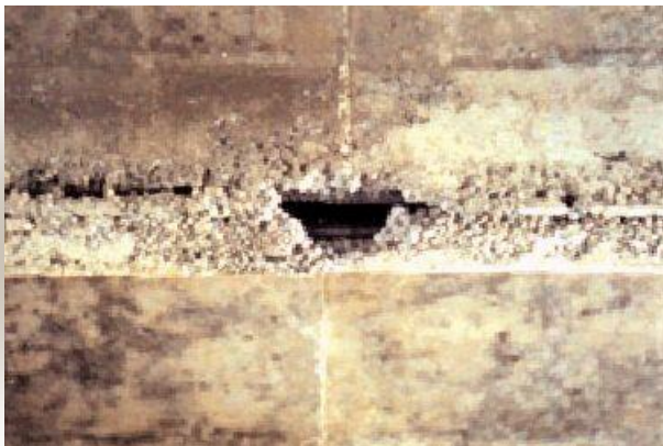
Figure 1-18: Honeycombing occurs when coarse aggregate separates from the mortar portion of the concrete.
