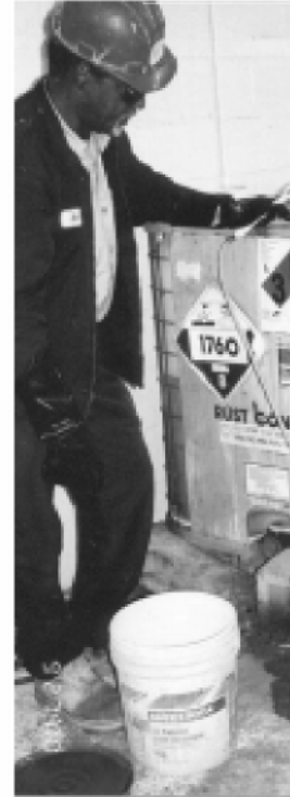
Figure 4-1: A CDP's Personal Protective Equipment (PPE) includes a hard hat, safety goggles or glasses, hearing protection, and gloves.
