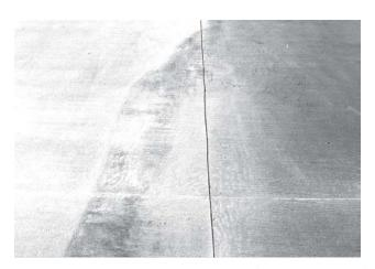
salts through evaporation or hydraulic pressures. The water evaporates and leaves a salt deposit on the surface.
