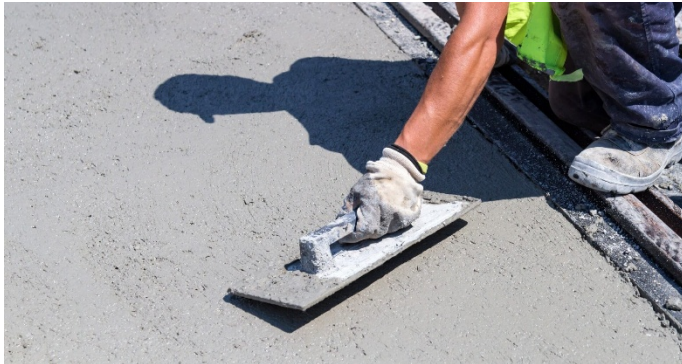
Example of Finishing Concrete
