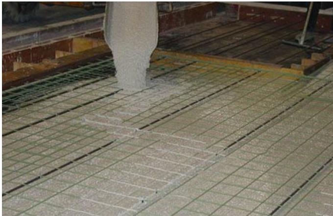
Placement of SCC
