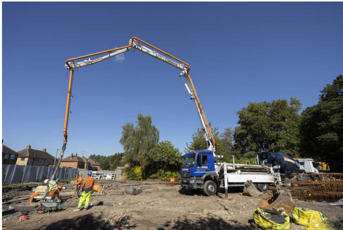
Example of pumping concrete
