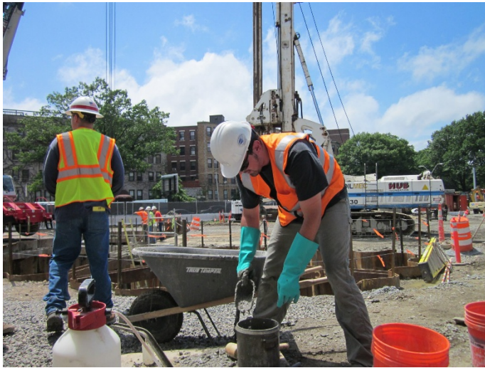
Example of On-Site Concrete Field Testing
